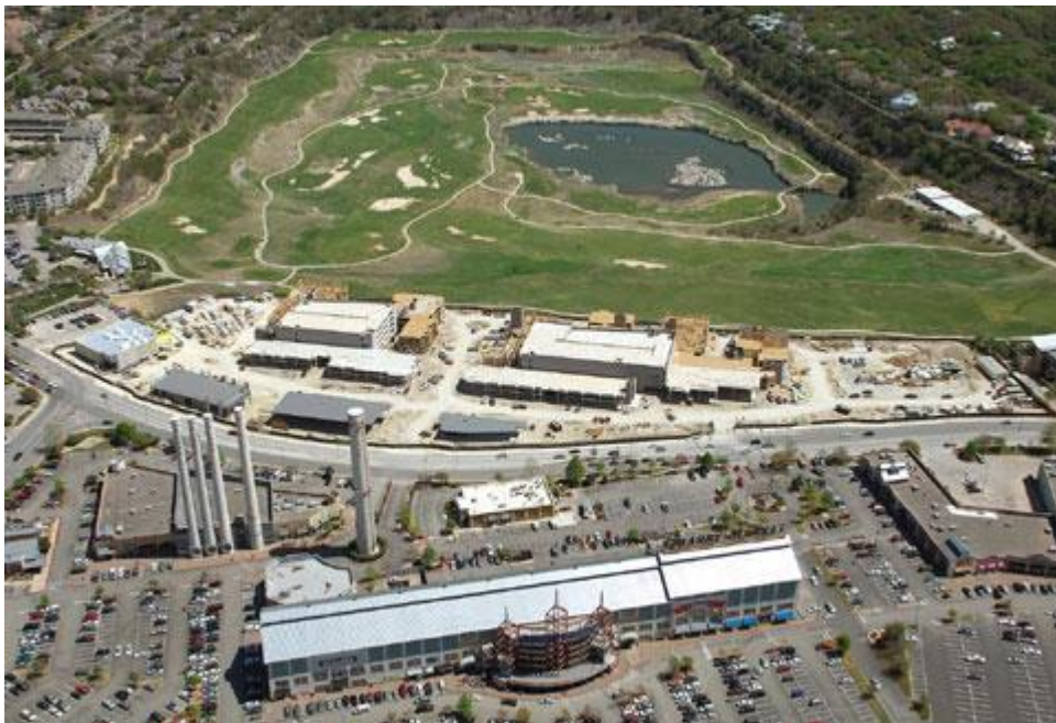
The Quarry Village is under construction near the Quarry Market.
